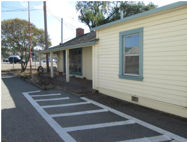
Photo 1: View of Building 1, looking east.
