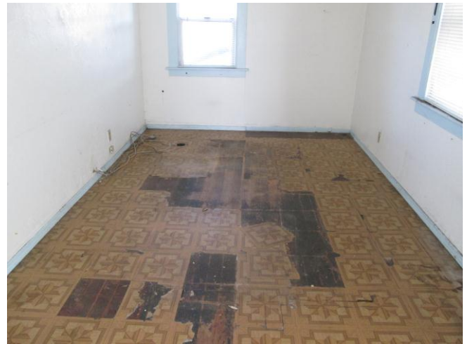
Photo 2: View of the interior of Building 1.
