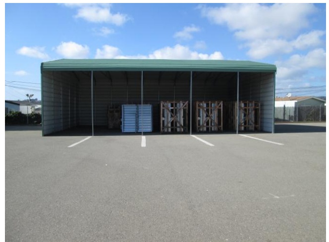
Photo 6: View of Building 4, looking west.
