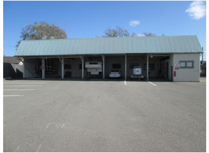
Photo 8: View of Building 6, looking east.
