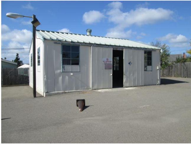
Photo 7: View of Building 5, looking west.
