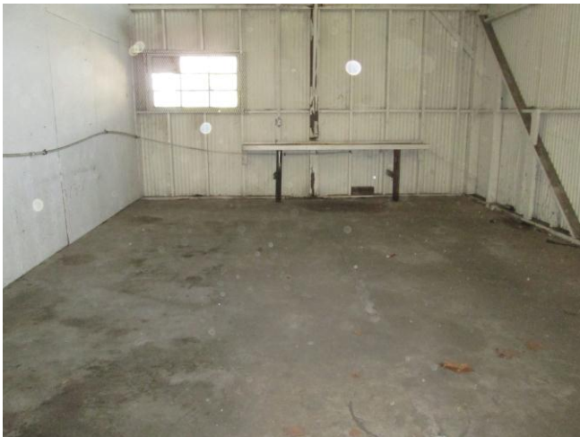
Photo 11: View of the garage area of Building 6.
