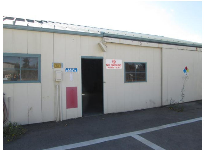
Photo 4: View of Building 2, looking south.
