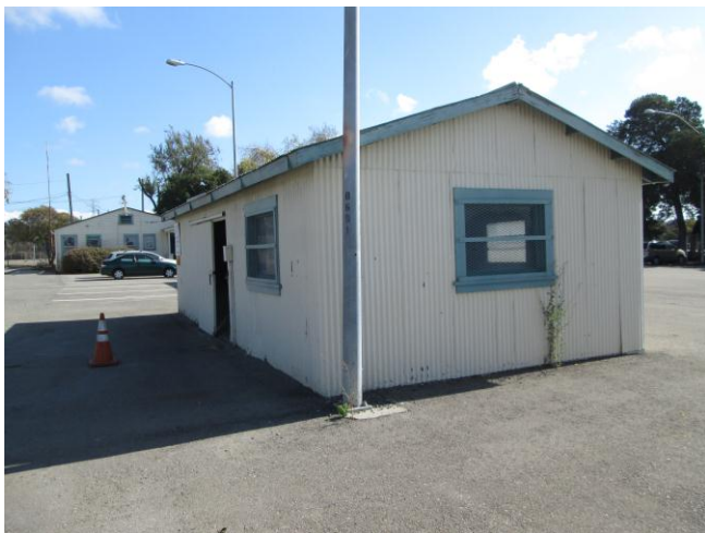
Photo 5: View of Building 3, looking east.
