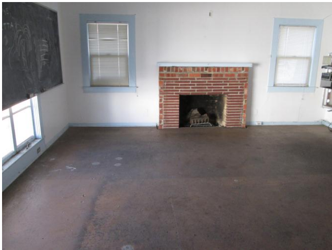
Photo 3: View of the interior of Building 1.
