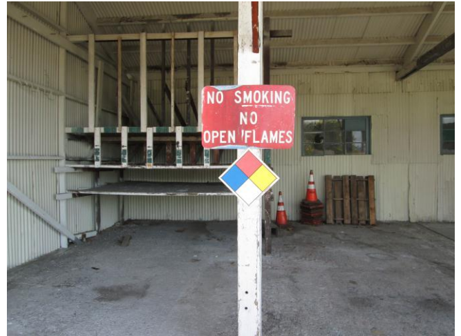
Photo 10: View of the garage area of Building 6.
